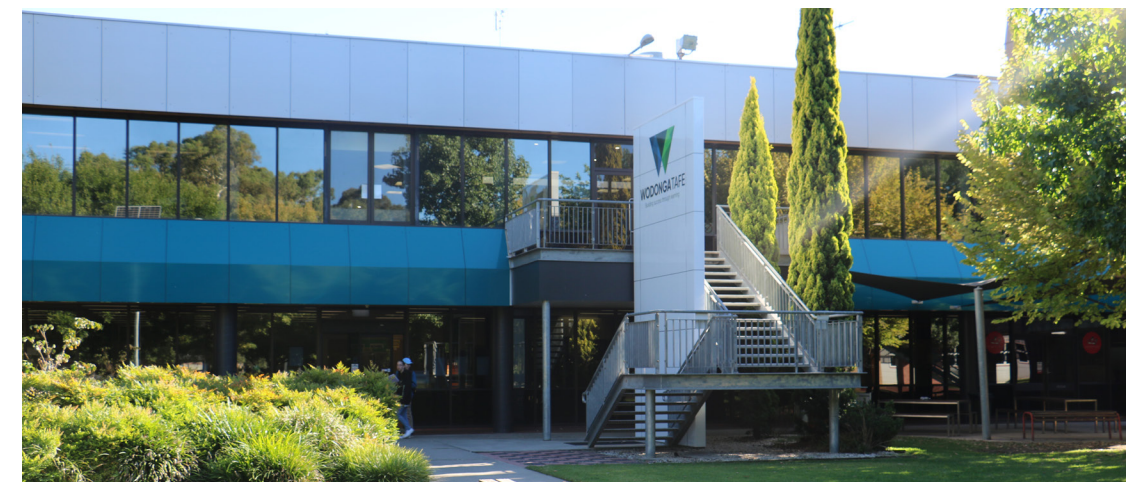
Entrance to Wodonga TAFE Building A, level 2. Photography Credit: Wodonga TAFE
